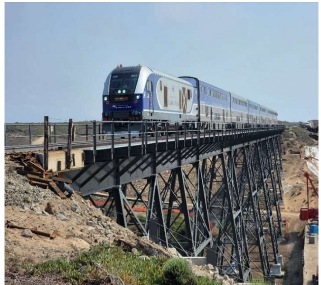
Narlon Bridge Replacement, Source: UPRR
