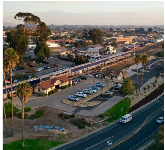
Grover Beach Station Expansion, Source: City of Grover Beach
